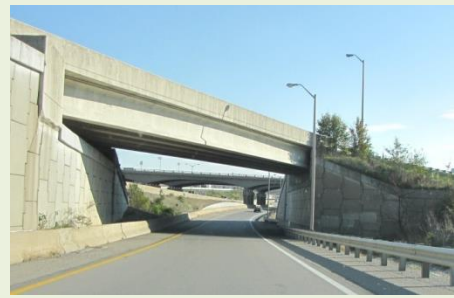
Image 1: I-75 SB Exit Ramp at US 42 Overpassing C/D Road to I-75
